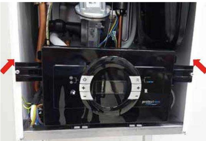
➤ Unscrew 4 screws holding side panels, bottom chassis, and the main housing.
