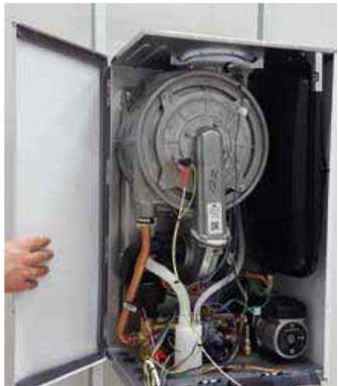
➤ **Dismounting Control Panel:** Detach the connecting terminal of the room thermostat, and ignition and ionization cables Mounted to the notches on the control panel. Open the cover by unlatching the notches of the control panel.
