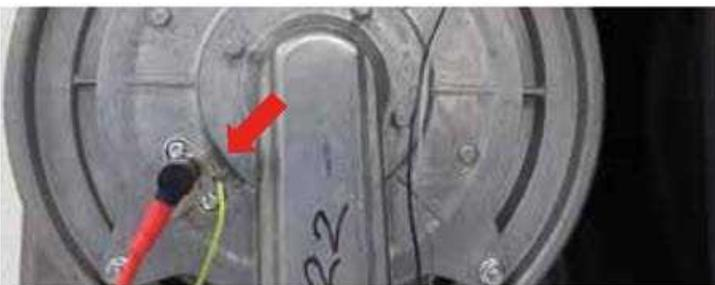
**NOTE:** When mounting the electrode, you must hear the locking sound as "click".
