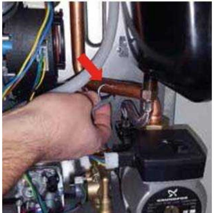
**Dismounting/ Mounting condensate trap and condensate trap hose:**
